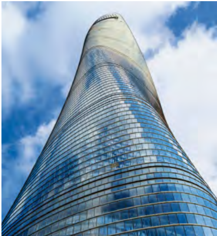
SHANGHAI TOWER – SHANGHAI, CHINA
